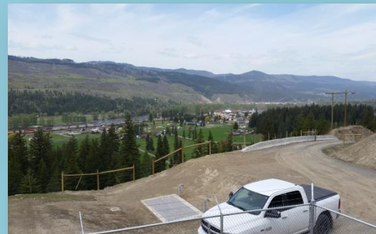
View from New Reservoir
