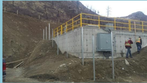
New Reservoir Construction
