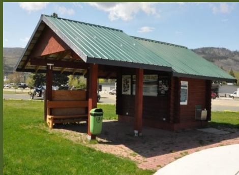
Splash Pad Shade Structure
