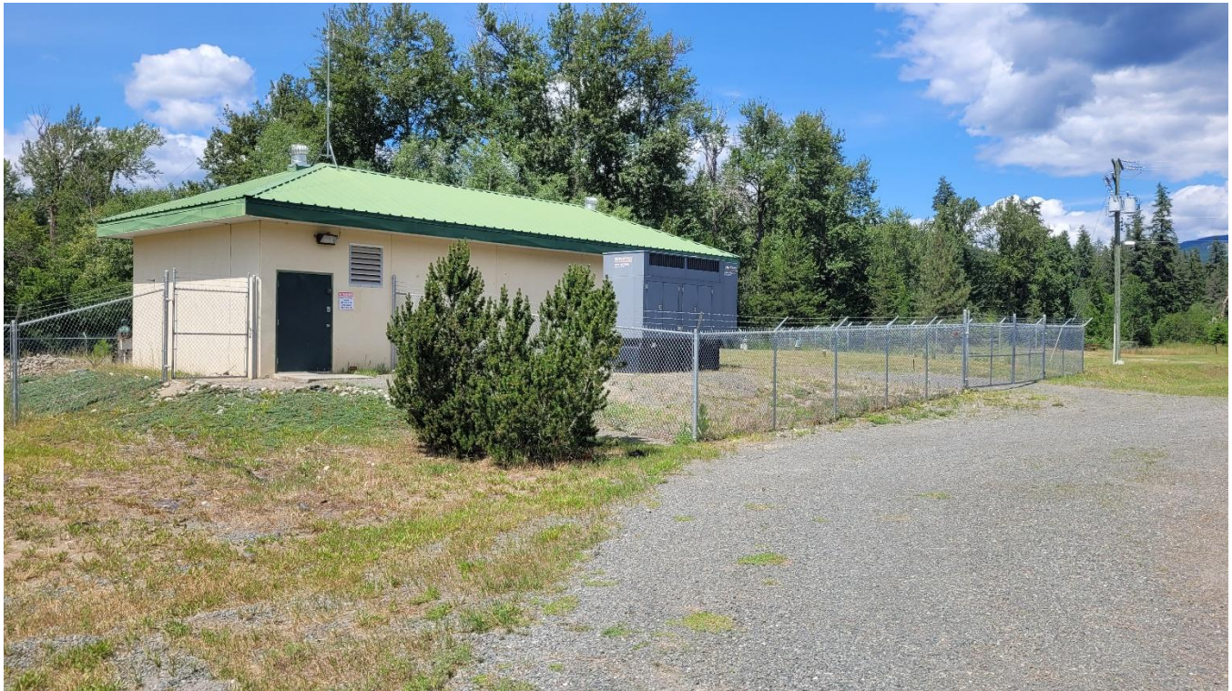
Community Water Plant – Spruce Crescent
