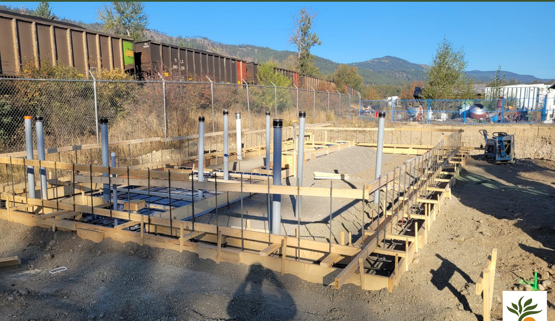
Filter Building Location
